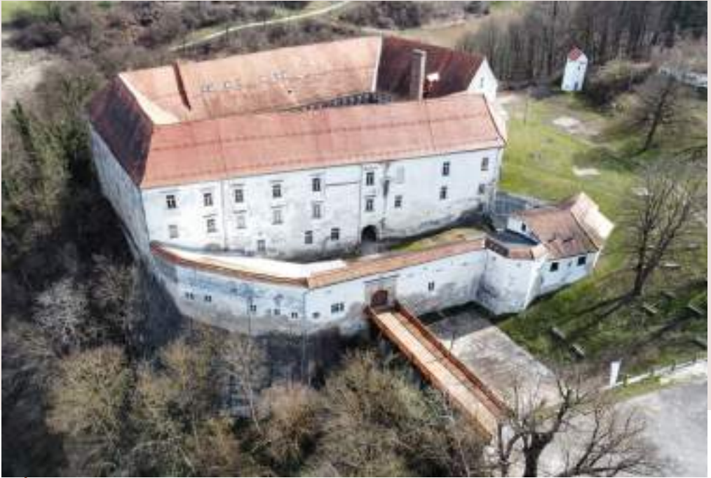
Aerial view of Cmurek Castle from the west (Photo: © Leon Friš)
