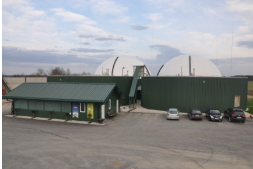
Figure 4: Biogas plant Keter Organica Gjerkeš 1. /4/
